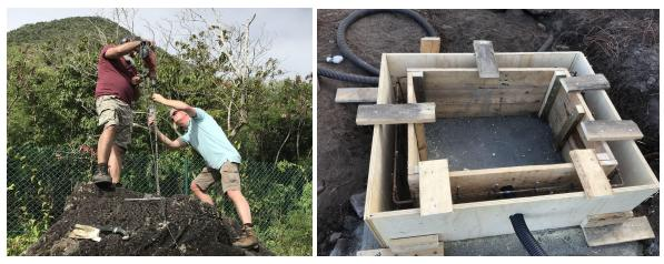
Fig. 2: Drilling for the GNSS monument (left) and construction of the housing for the seismometer (right).
